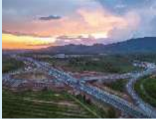
Phnom Penh - Sihanoukville Expressway Project, Cambodia
