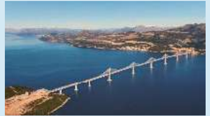
Peljesac Bridge, Croatia
