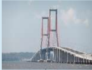
Suramadu Bridge, Indonesia
