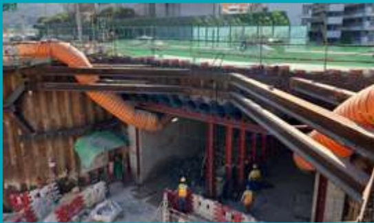
Horizontal Pipe Piles and Trenchless Excavation - Shek Mun - CV/2020/02
