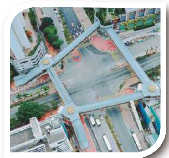
CEDD Contract: KL/2016/01 – West Kowloon Reclamation – Main Works (Remainder) – Footbridge at Junction of Sham Mong Road / Tonkin West in Sham Shui Po
