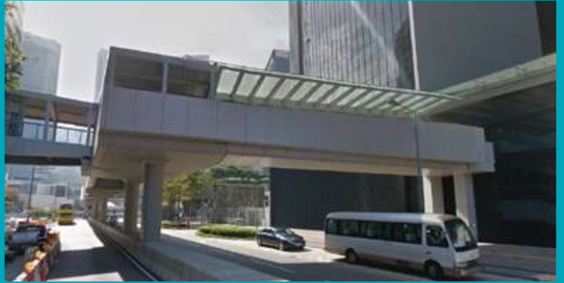
Structural Steel Footbridge - Admiralty - HY/2013/13
