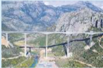
Bar-Boljare Highway, Montenegro
