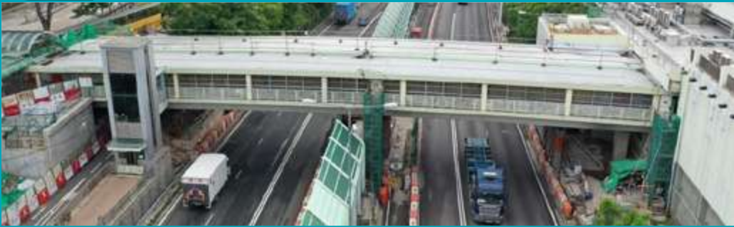
Prestressed Concrete Footbridge - Fanling Station - CV/2016/06
