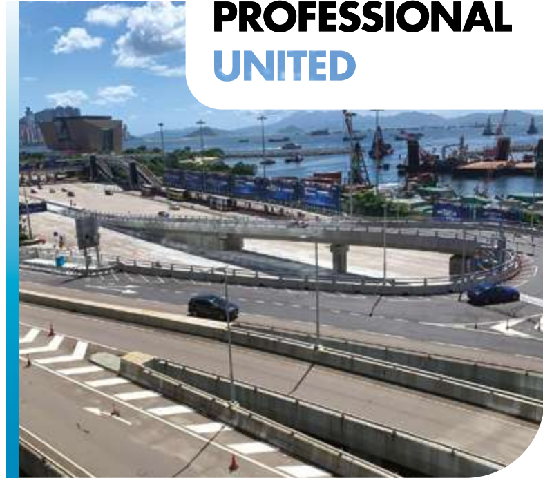
Road Improvement Works in West Kowloon Reclamation Development
