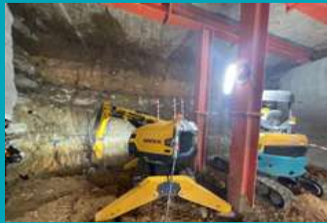
Horizontal Pipe Piles and Trenchless Excavation - Shek Mun - CV/2020/02
