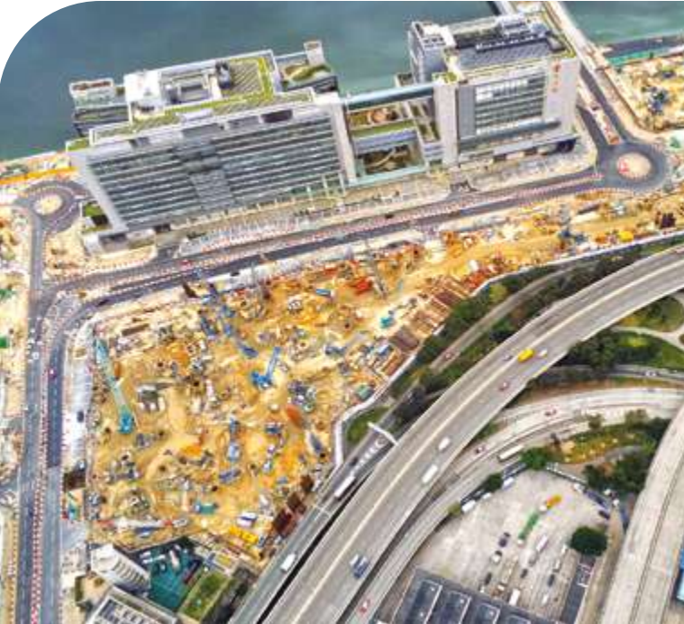
New Acute Hospital at Kai Tak Development Area
